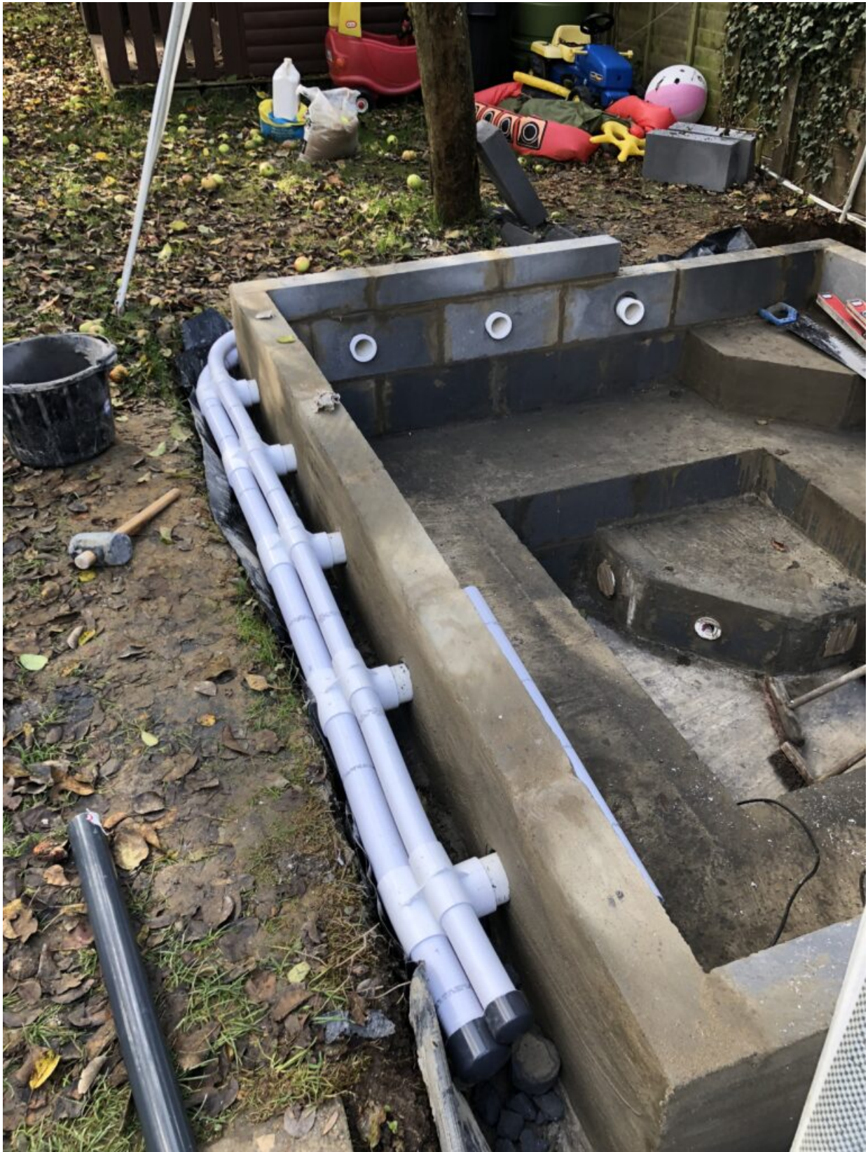
Pipes in for Hot Tub
