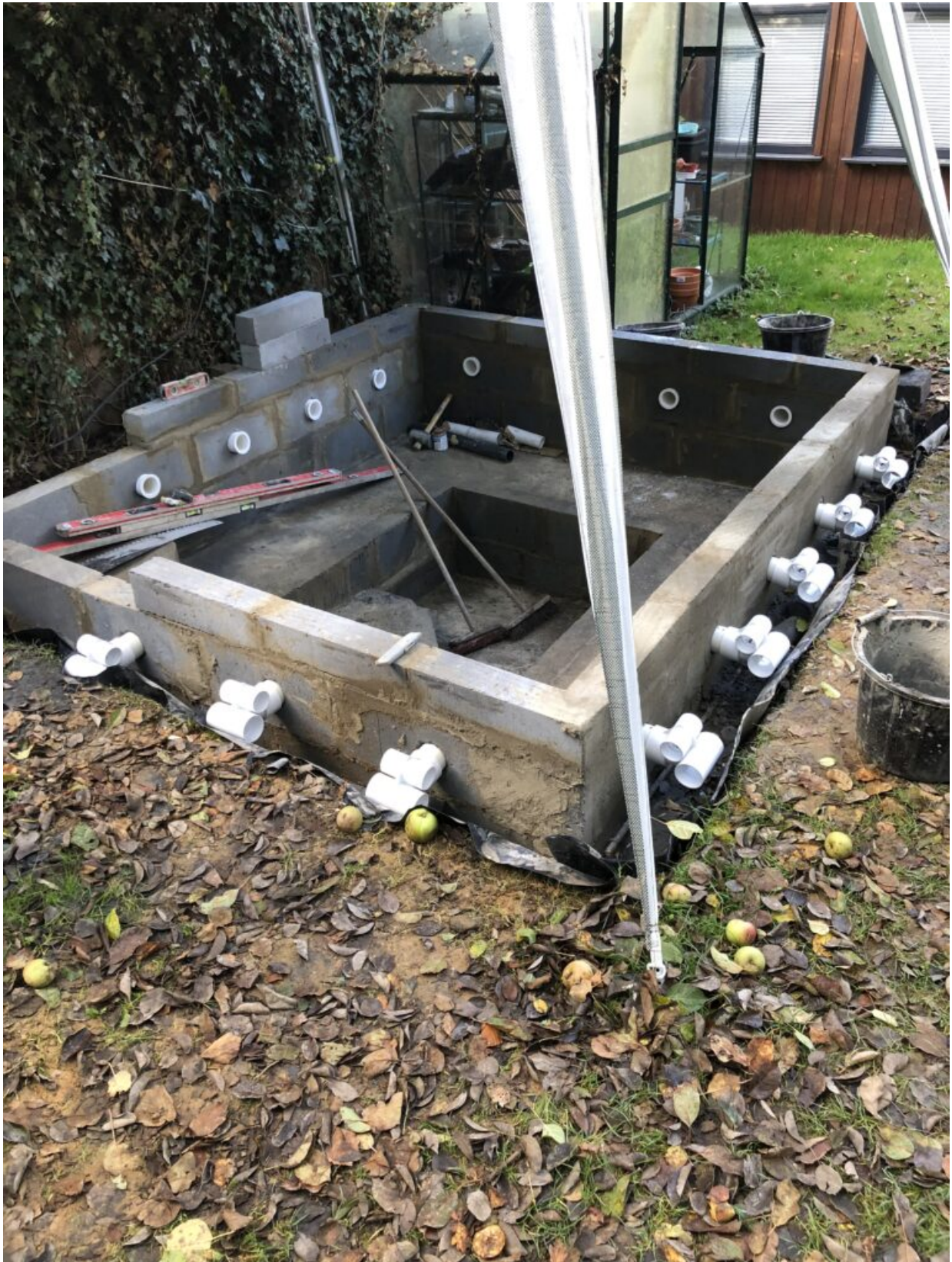
Plumbing in for hot tub
